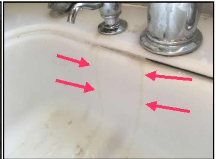
aging kitchen faucet leaking
